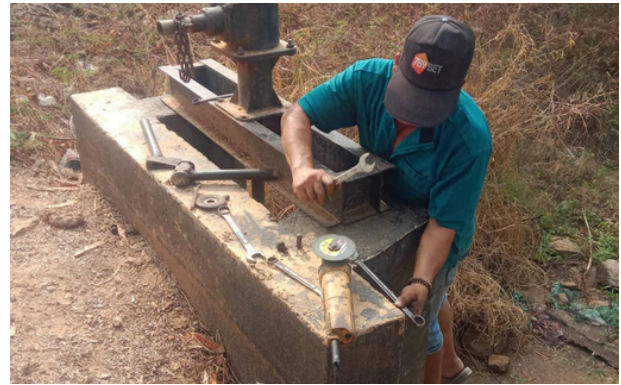
Infrastructure maintenance: Replacing a broken water gate in Banteay Neang Commune, 2024 ©Nurture Project
