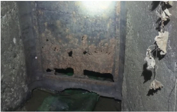
Technical inspection of water gate functionality in Banteay Neang Commune, 2024 ©Nurture Project
