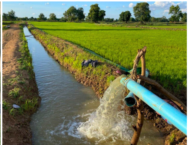
Sub-canal irrigation supplied by a solar pumping station in Peam Village, Kdol Tahean Commune, Bavel District, 2024 ©EGE Cambodia
