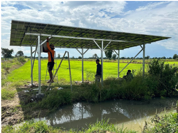
Deep-well solar panel installation for irrigation in Peam Village, Kdol Taken Commune, Bavel District, 2023 © EGE Cambodia
